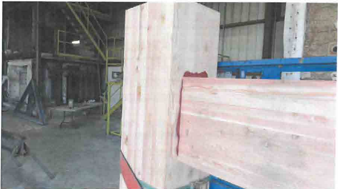
Figure A-4. Typical Beam and Column Connection.
