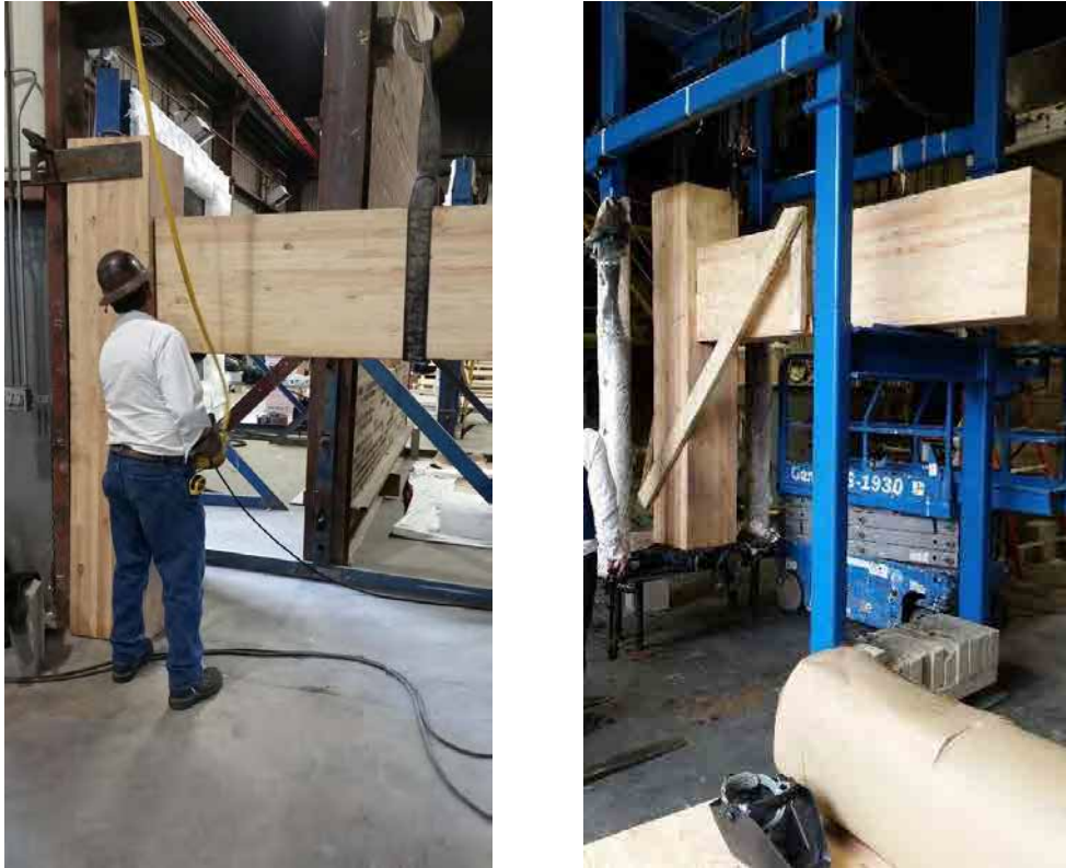
Figure 1 – Test specimen being assembled, before CLT floor is installed
