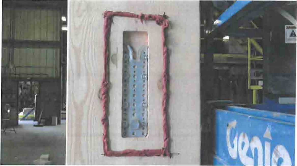
Figure A-3. Column Prepped.
