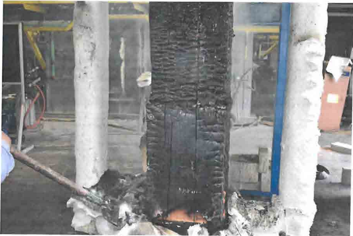
Figure E-6. Base of Beam after Fire Exposure.
