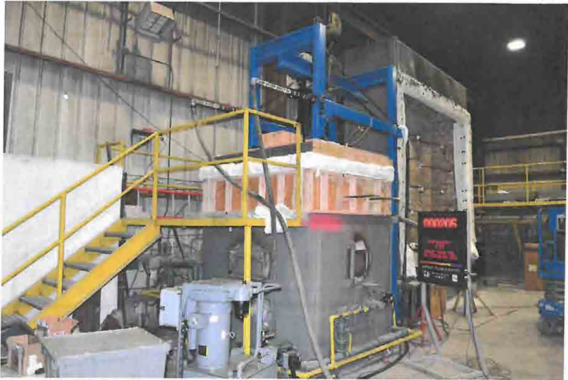
Figure E-1. View of the Assembly and Applied Load Equipment at 2 min 5 s.
